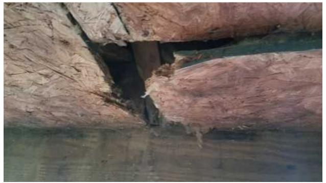
Wood: "First" wood untreated, too close to earth (8" or less) is prone to rot carpenter ant and especially termite damage as discussed. Repair/treatment is recommended to deter/stop termite activity
