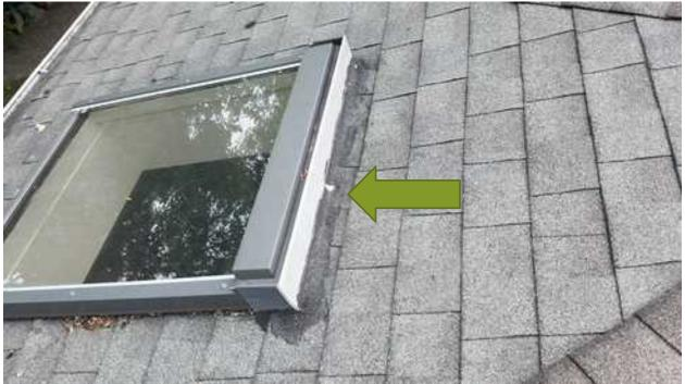
3C.03 Shingles, asphalt: eroded/pitted/granules missing is consistent with the aging process of an older roof. Recommendation: Monitor, repair and budget for future functionality Multiple layers and darker colors of roofing will adversely affect roofs longevity of require additional ventilation, etc
