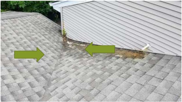
Vinyl/aluminum wrapping, soffit and or siding loose/missing/damaged/bulging in many areas.
