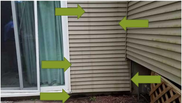
Vinyl siding deforming/melting (exceeded 160 degrees?) on the left side perhaps from outdoor grill, electrical malfunction (excessive heat) or other heat source that was too close or defective. Recommendation: Remove siding and assess. This is a safety concern
