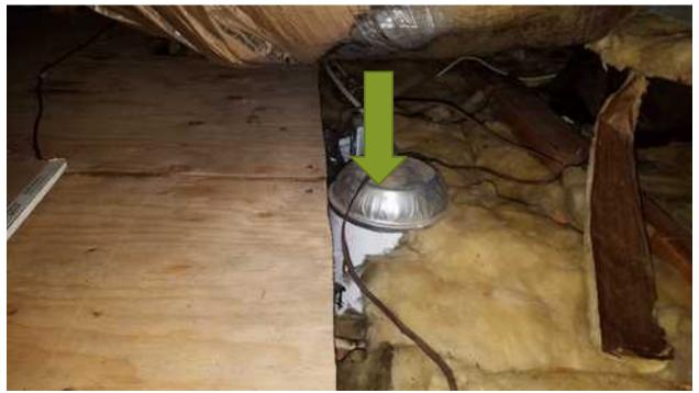
5C.77 Light fixture loose (hanging from wires)/broken outside at the rear. Recommendation: Replace
