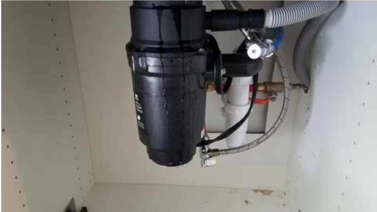
4C.07 Ejector pump area odor in laundry room may not be properly vented/sealed. Repair is recommended
