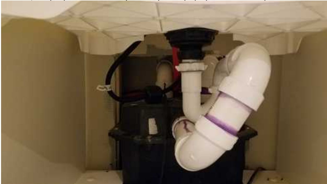
4C.07 Ejector pump area odor in laundry room may not be properly vented/sealed. Repair is recommended
